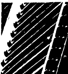
A closeup shows a few of the 5,064 glass tubes that form the solar collector for the building. The tubes are arranged in 211 modules of 24 tubes each.
