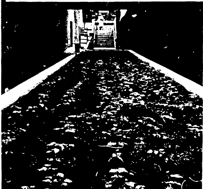
A closeup shows a few of the 5,064 glass tubes that form the solar collector for the building. The tubes are arranged in 211 modules of 24 tubes each.
