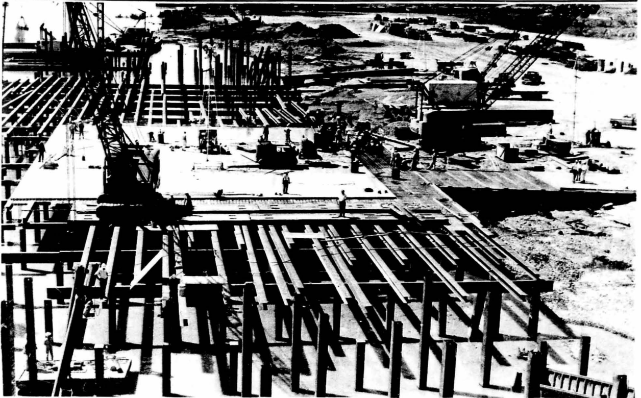
ABOUT 75 MILES OF PILING ARE BEING DRIVEN AT NEWPORT NEAR SAIGON AS PART OF U.S. CONSTRUCTION EFFORT.
