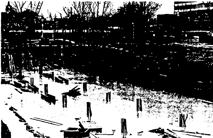
CLASSROOM BUILDING APPEARS TO BE SWIMMING POOL UNDER CONSTRUCTION
