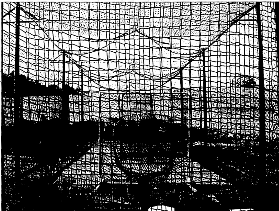
The new four-tunnel hitting complex was completed just in time for a week-long baseball camp. The complex sits adjacent to Abe Martin Field. TED SCHURTER DAILY EGYPTIAN
