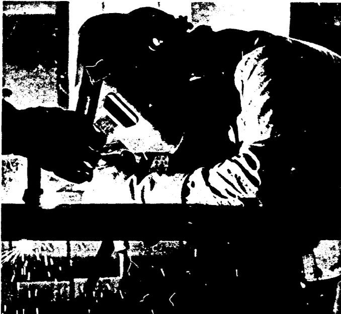
Arch Walbright, above, welds sections of pipe to be used for plumbing. Dick Null, right, wraps insulation around pipes on the second floor.
