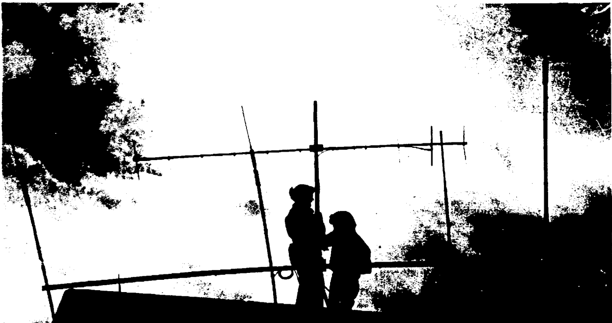
Members of the SIU-C Amateur Radio Club check the club's antennas located on top of the roof of Technology Building D for loose cable connections.
