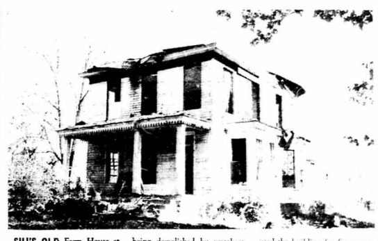
SIU'S OLD Farm House at 1311 South Thompson street is being demolished by wrecker's. The agriculture department has used the building for five years.
