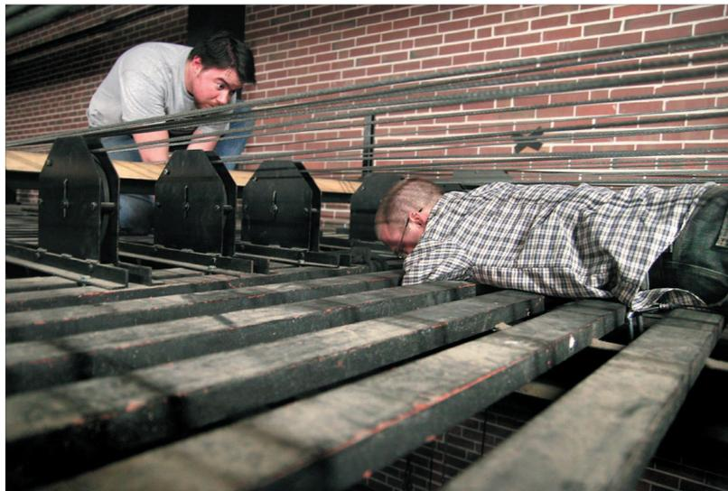
**ABOVE:** Stephen White, left, and Jeff West, graduate students in technical directing, lower lights and pieces of an old set from the grid above McLeod Theater's stage Monday. The grid is 52 feet above the stage and houses pulleys and steel cables that allow scenery and curtains to be raised and lowered.
