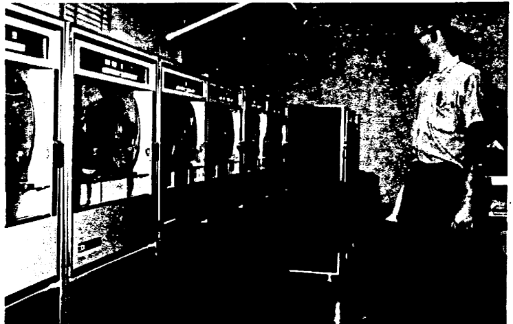
STUDENT WORKER MIKE BARTLETT CHECKS SOME OF THE EQUIPMENT AT THE DATA PROCESSING AND COMPUTING CENTER.
