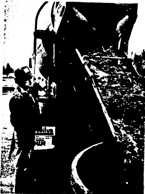
Carry Picket, one of the workers on the construction site for the SIU-C Law School building, prepares a mix of concrete that will be used in installing the new 7-inch steam pipe system for the building.
