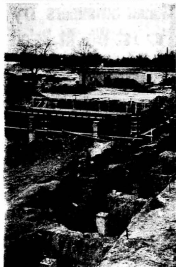
A sectional view of part of the central wing of Southern's new Agriculture building shows a row of floor-supporting reinforced concrete pillars near
