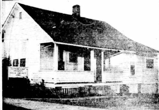
Old frame houses being used for classrooms and offices
