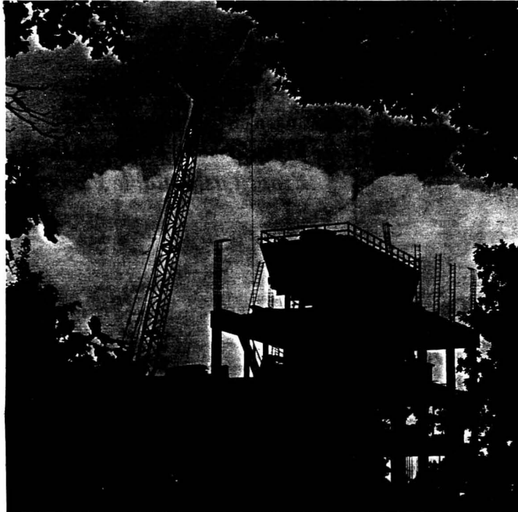
CHANGING SKYLINE—The progress of construction continues to change the skyline of the Carbondale Campus. Here, framed by nearby trees, is the Physical Sciences Building south of the University Center. (Photo by John Baran)
