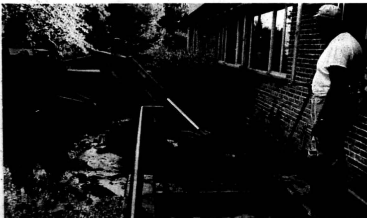
Workmen clear mud from Felts Hall
