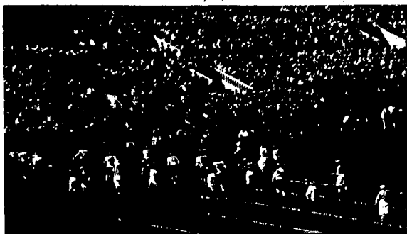
EVERYBODY SEEMS to be heading toward the sidelines in this unusual shot taken from the top of the new power plant.
