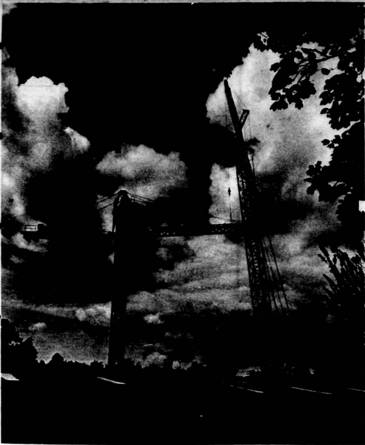
New crane now at work
