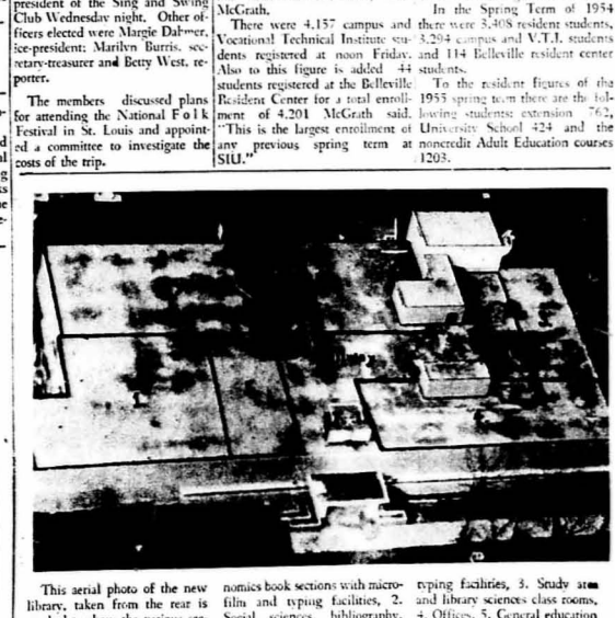
This aerial photo of the new library, taken from the rear is marked to show the various sections of the building. 1. Business administration and economics book sections with microfilm and typing facilities, 2. Social sciences, bibliography, public catalog, microfilm and typing facilities, 3. Study area and library sciences classrooms, 4. Offices, 5. General education book section.
