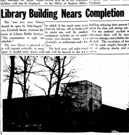
The new 2-story library building is nearing completion. Students will have access to 42% of the building when it is opened, and as work continues this percentage will increase.
