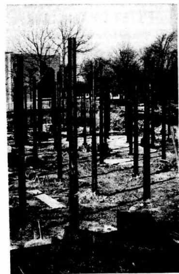
Shown above is the new 1953-54 winter quarter. Library construction during the
