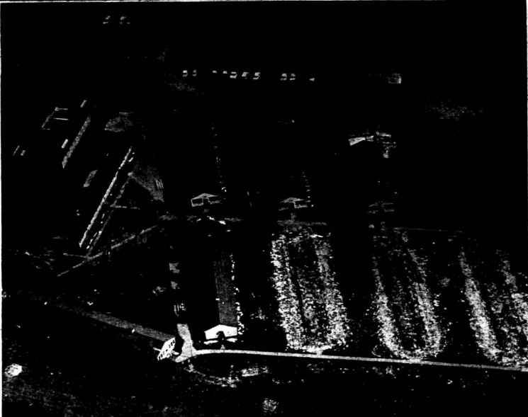
DISAPPEARING DOWDELL - Dowdell Halls, a group of barracks buildings brought to SIU from Camp Ellis, Ill., in 1951 to serve as "temporary" dorms for men finally are being removed to make way for the new $10.5 million University Park Housing Development. However, they aren't going into the junk heap. Three will be used by the Illinois Youth Commission forestry camp near Anna and the others will be moved to the SIU camps on Little Grassy Lake.
