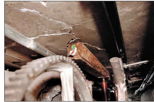
A piece of wood supports part of a falling ceiling in one area of the nearly seven-mile-long underground tunnel system that connects buildings around campus. Amaro said the ceiling, which is deferred maintenance, is not hazardous but needs repairing.
