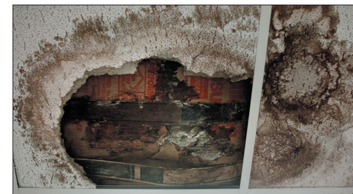
Water damaged tiles, like this, plague the Agriculture Building. These tiles can be found in many other buildings around campus including the Blue Barracks and Faner Hall.
