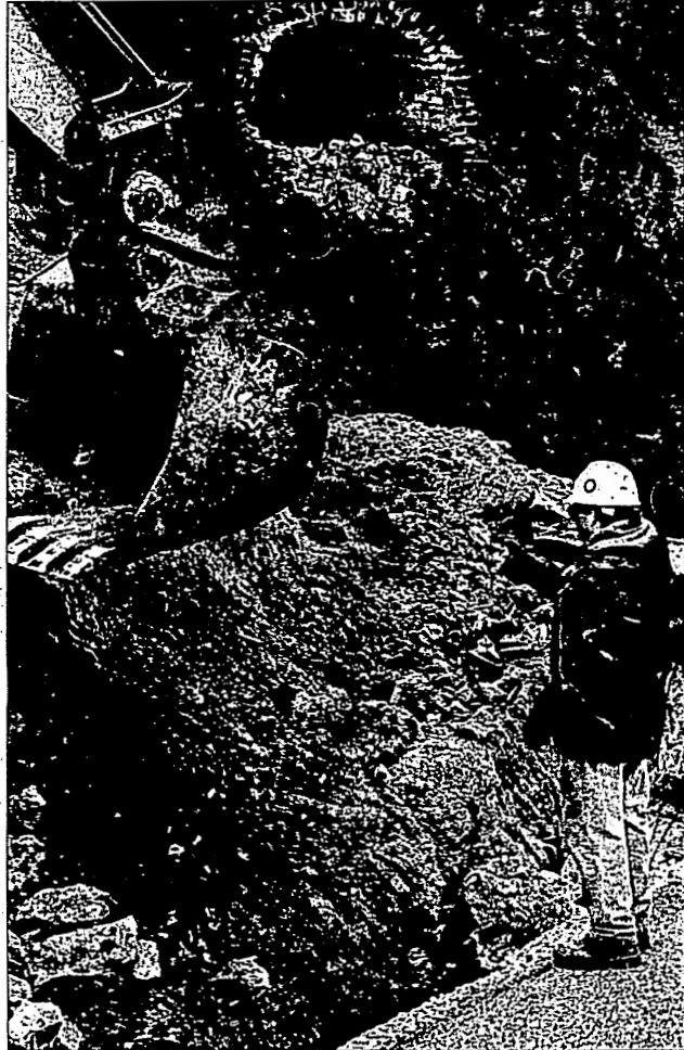
Robb Pratt, assistant project supervisor from Streator, directs a backhoe behind Altgeld Hall on Wednesday afternoon. Pratt works for Janko Building Company, which is constructing the new addition to the hall.
