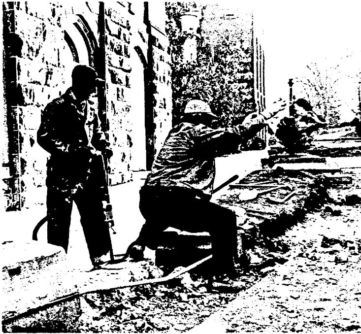
NEW LOOK FOR THE OLD CAMPUS—Demolition of a drive that once cut through the "old" campus is now under way. The drive leading from the Old Main gate is being broken up and the area will be
