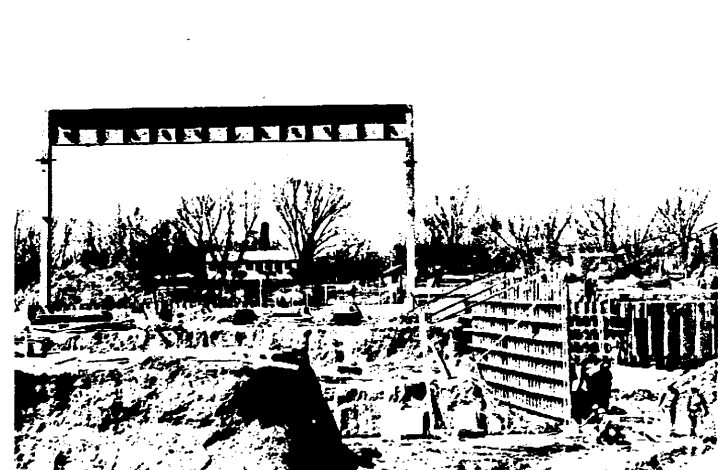
THE STEELWORK WILL ONE DAY REPRESENT THE ARCH SU'S "GRAND THEATER" IN THE NEW COMMUNICATIONS BUILDING.
