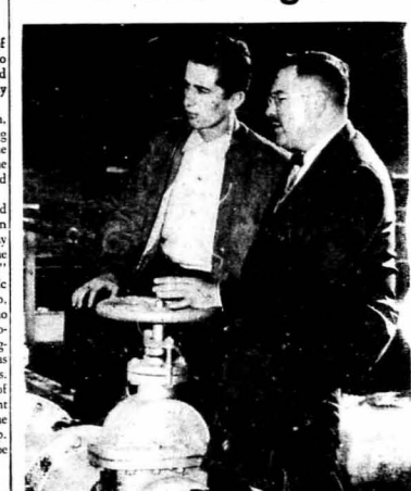
Robert E. Walker, (left) first SIU public health major, and Tony Favro, sanitarian, inspect the facilities at the Carbondale sewage disposal plant.
