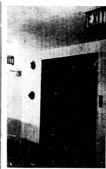
THIS IS SOUTHERN'S first elevator and it is located in the new Life-Science building. Students will not have access to the elevator though, since it will be used mainly for maintenance purposes and for transporting heavy equipment. Part of the extensive fire alarm system is next to the elevator. The building is built completely of steel, brick and cement and fire-proof throughout.
