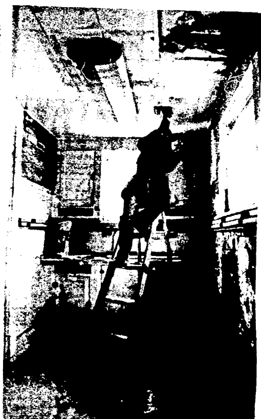
Yolanda Tullar removes ceiling tiles to retrofit the house for the Shawnee Solar Project.
