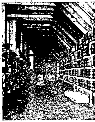
After the library was condemned, 75 percent of the books had to be stored in various spots about the campus. Above, the attic of the library building becomes a storage space for the overload.
