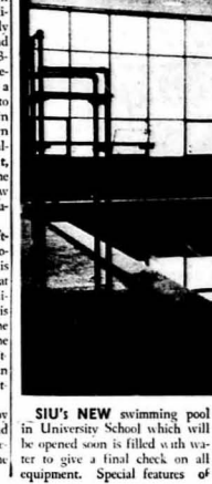
SIU's NEW swimming pool in University School will be opened soon. It is filled with water to give a final check on all equipment. Special features of
