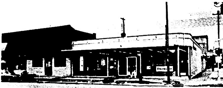
Where Walnut Street meets Illinois Avenue (foreground) will be the northeast corner of the parking garage and hotel site.
