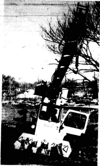
When Doc Allen came to work Monday morning, he found the situation sticky. Last week's rain left his crane in mud up to the axles at the construction site for the recreation building on Grand Avenue. (Staff photo by Jim Cook)
