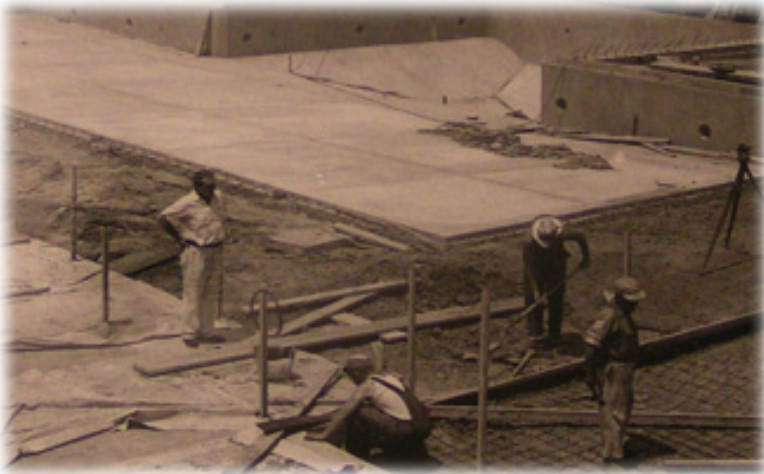
Photograph 2: Building of the Herrin Swimming Pool mid 1950s. Photograph courtesy of the Herrin Public Library and Herrin City Historical Society.
