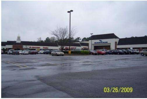
Figure 7. Example of a typical commercial development in Raleigh, NC.
