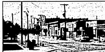
The Washington Street improvements between Jackson and Oak Streets were recently completed. The project involved the installation of planting islands, brick pavers along the edge of the sidewalk, and decorative lighting like that in the Town Square area.
