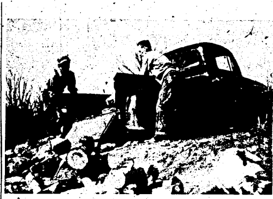
WILLIAM MACDONALD, left, and Jim Miller, APO pledges, unload a truck load of rocks which were dumped along the creek bank at the bridge site, in order to help prevent erosion and avoid a bridge washout. The rocks were taken from an old farm house basement near the picnic area.
