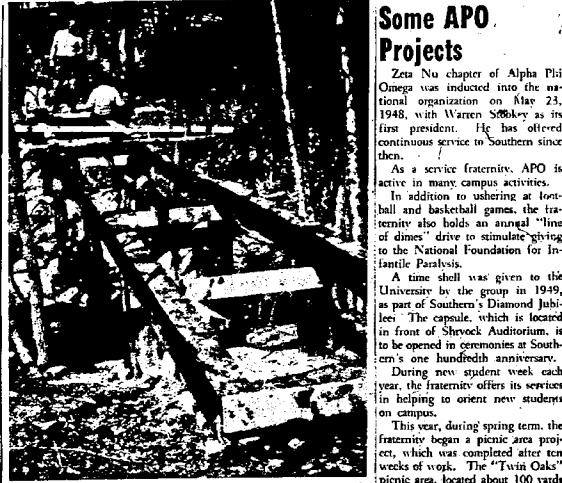
APO MEMBERS began cutting the bridge, after all the superstructure has been put securely in place. Service fraternity members worked on the project week-ends only, and completed it in about ten weeks during spring term.
