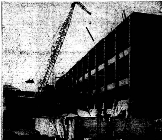
RIISING HIGH The Home Economics building continues to grow daily. The size of this section is illustrated by the workers which appear as midgets against the facade. Enough funds are available right now to complete the outside shell of the building.
