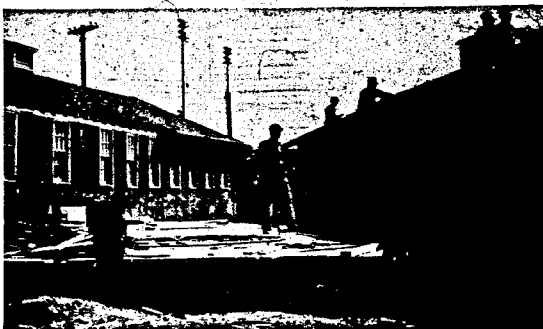
PHYSICAL PLANT workers as they began construction early this week on the addition to the Student Center which will connect the Center with the Post Office building.
