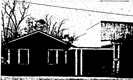
THE NEW barracks annex to the university cafeteria. The physical plant is now working on the interior of the annex which will open into the regular cafeteria building.
