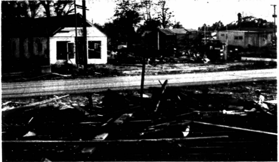
On April 27, a tornado hit the small Southern Illinois town of Thompsonville, damaging and destroying property as well as scattering debris throughout the area. Clean-up is complete, but many Thompsonville residents are now facing the job of rebuilding their community (Photos by Dave Butler)
