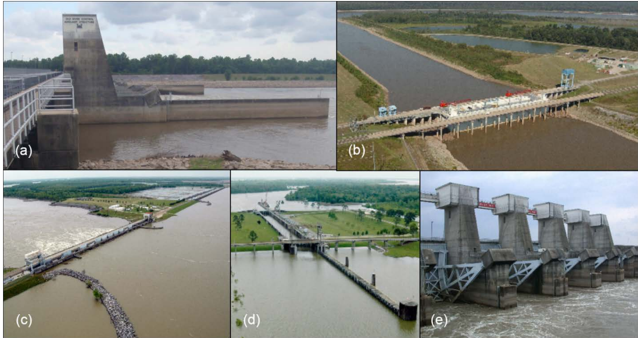
Figure 2.3. Photographs showing: (a) the auxiliary control structure, (b) the S. A. Murray, Jr. Hydroelectric Power Facility (U.S. Army Corps of Engineers, New Orleans District 2009), (c) the low sill control structure and overbank structure (U.S. Army Corps of Engineers, New Orleans District 2009), (d) the Old River Lock (U.S. Army Corps of Engineers, New Orleans District 2009), and (e) the auxiliary structure (U.S. Army Corps of Engineers, New Orleans District 2009).
