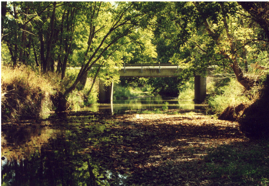
Figure 10. Big Creek upstream fish monitoring station (IEPA code IXJ-02), 7 September, 2000. Above bridge, looking downstream.
