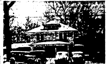
The building shown above is the newly acquired Agriculture building. This building, located at 1028 S. Thompson, was recently put into use, but is still undergoing repair.
