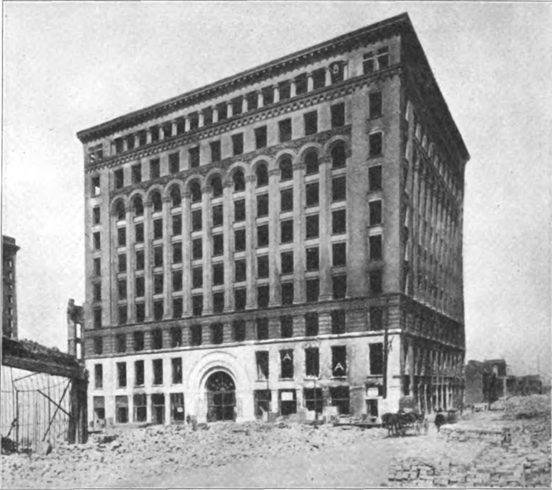
A BRICK BUILDING WHICH HAS WITHSTOOD INTENSE HEAT. 5095 The brick and terra cotta walls are virtually unscathed.
