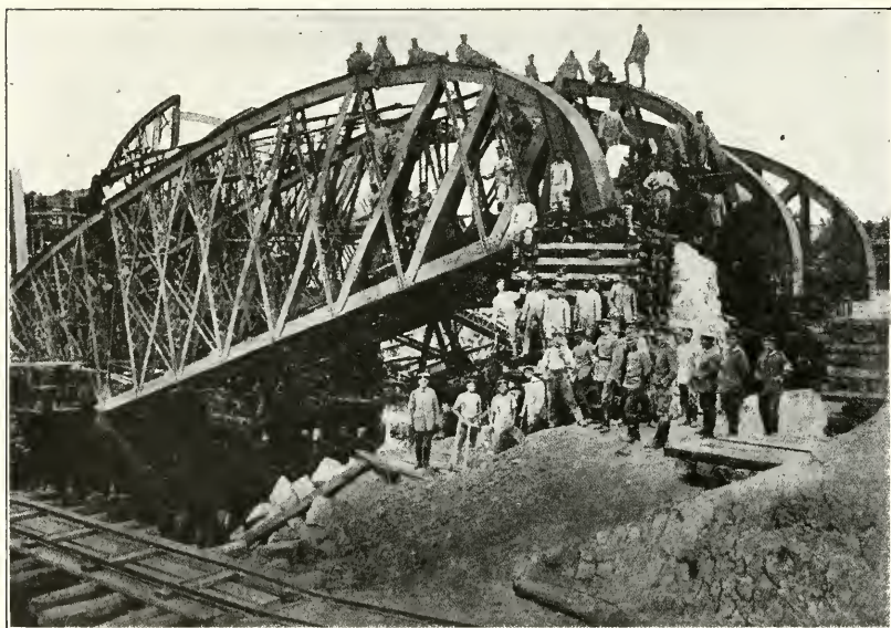
GERMAN PIONEERS RECONSTRUCTING A BRIDGE IN GALICIA.
