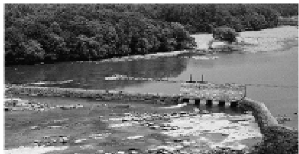
Figure 4. Low-head run-of-river dam on the Savannah River near Augusta, Georgia, a significant blockage for fish passage. Source: U.S. Library of Congress, Historic American Buildings Survey, Historic American Engineering Record.
