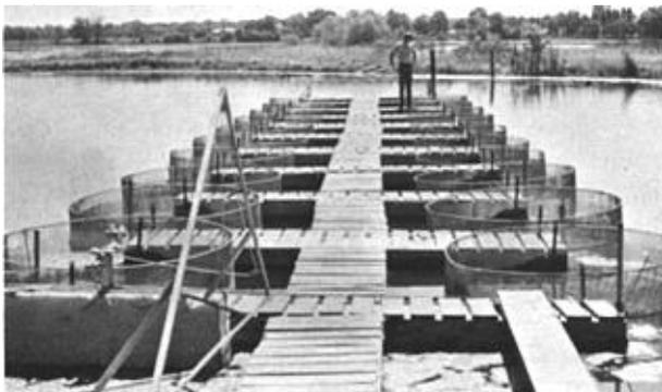
Fig. 2. Floating dock and cage system positioned in rearing pond.
