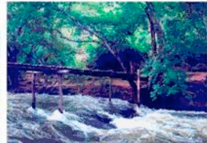
construction of wooden Bridge
