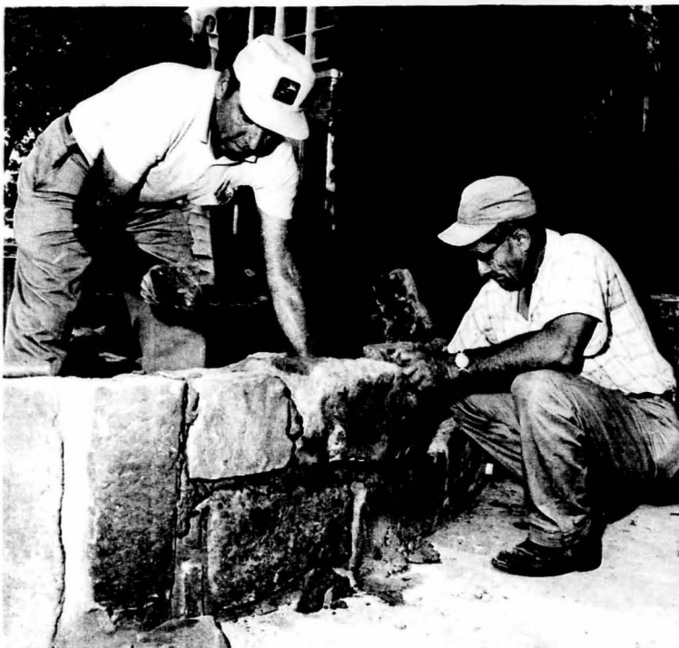
NEW PLANTERS --Two masonry planters are being installed in the space at the south end of Allyn Hall. Bricklayer Darrell Hodson, Harrisburg, (left) and Russell Mifflin, Murphesboro
