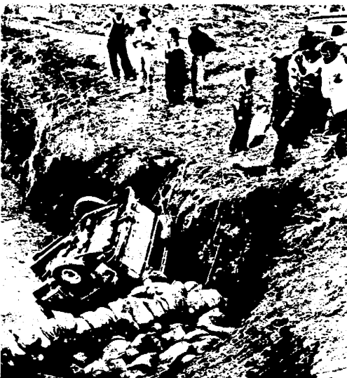
LAST-DITCH FIGHT — Floodfighters throw sandbags onto wire mat to block crevasse (lower right) in Rock Creek levee north of Quincy, Ill. (AP Photo)
