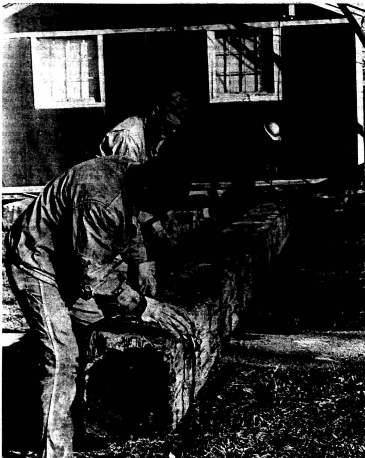
READY FOR MOVING- Workmen place a timber beneath the temporary building formerly used for biology laboratories as they prepare to move it a block south of its present location. Left to right are
