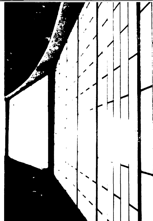
TRANSLUCENT PANELS ARE USED FREELY AROUND THE PERIMETER OF THE SIU ARENA. NOT ONLY IS THE ILLUMINATION EASIER ON THE LIGHT BILL, BUT THE OUTSIDE LIGHT PRODUCES THIS ORIENTAL EFFECT.
