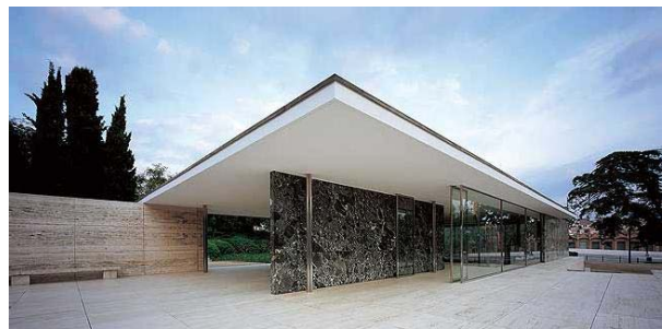
Figure 2.7. Barcelona Pavilion [Online Image]. Source: Pepo Segura.
