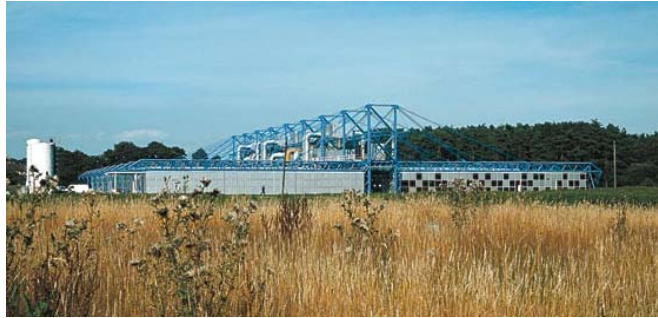
Figure 3.2. Exterior view of Inmos Microprocessor Factory [Online Image]. Source: richardrogers.co.uk/
