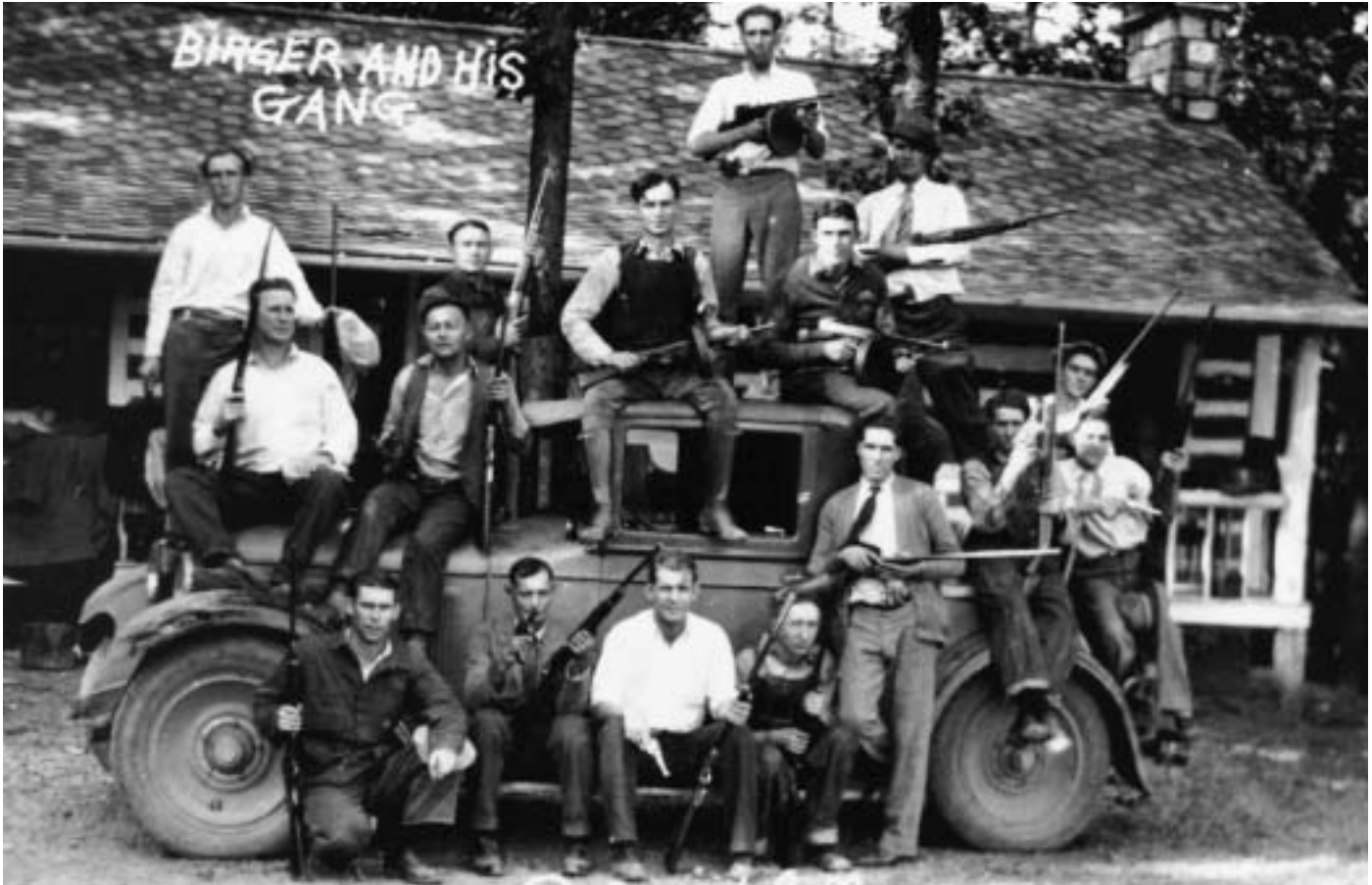
▲ Southern Illinois bootlegger Charlie Birger (center, sitting on car roof) and his gang at Shady Rest. Photograph courtesy of Gordon Pruett.
